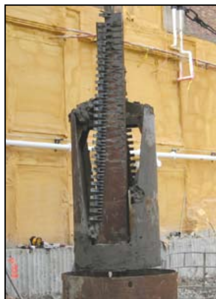
Machine being lowered in open shaft.
